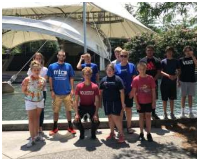
The youth of MCUMC and MTC served those in need of home repairs in Knoxville, Tennessee, during the July 2018 youth mission trip. (Photo provided by George Winterstein)
